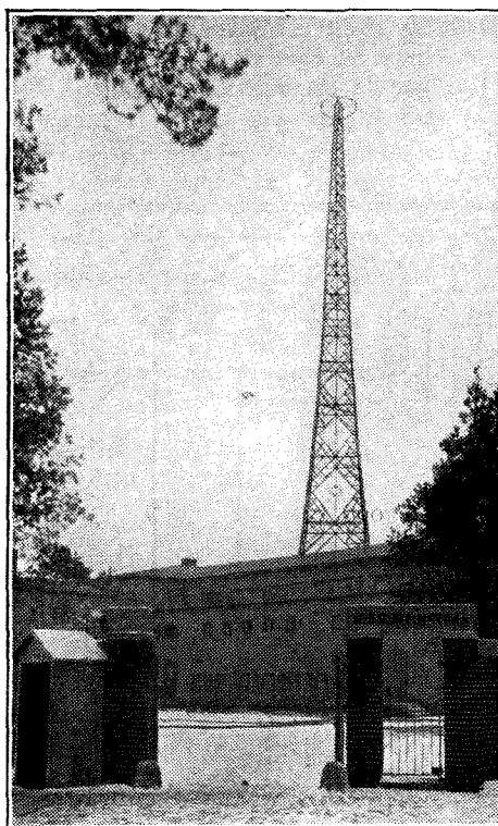
The "Deutschlandsender"—Berlin's 100-kW. station—with its anti-fading aerial.
