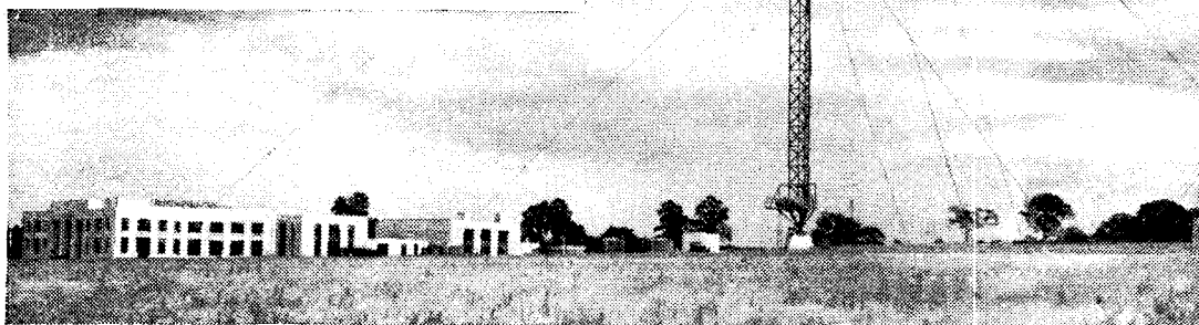
A general view of the B.B.C.'s new high-power station at Wychbold, near Droitwich, to be opened early in September.
